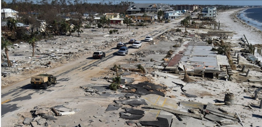
Hurricane Michael (2018) Mexico Beach, Florida
