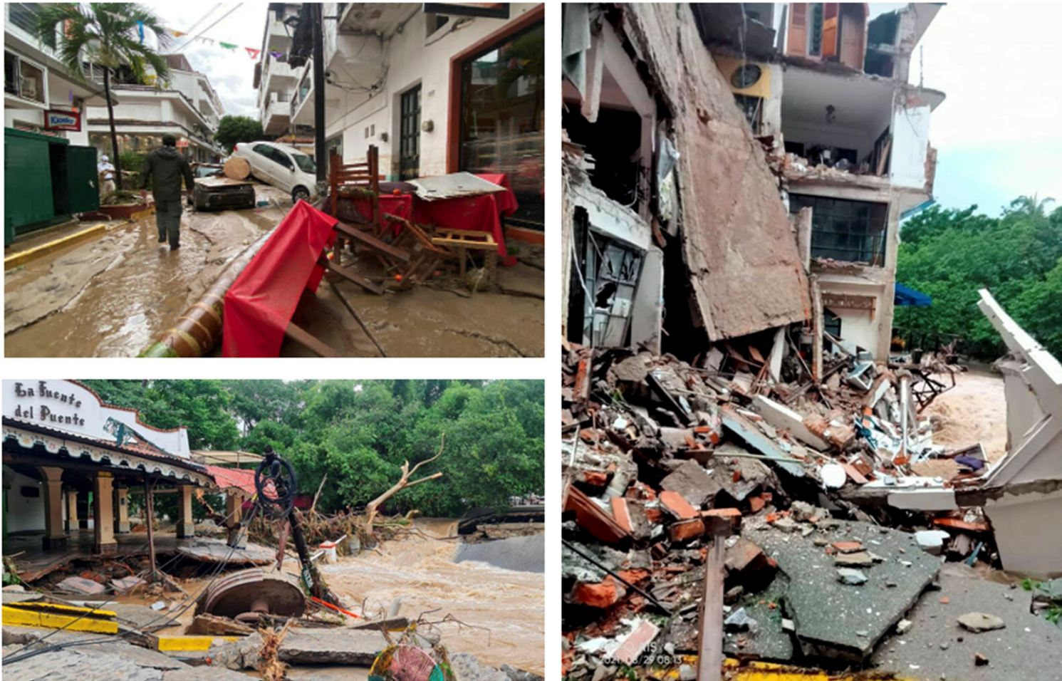
Figure 6. Select images illustrating damage associated with Hurricane Nora in Puerto Vallarta in Jalisco, Mexico, including the partial collapse of a hotel (right image) leading to one fatality. Images courtesy of Reuters.
