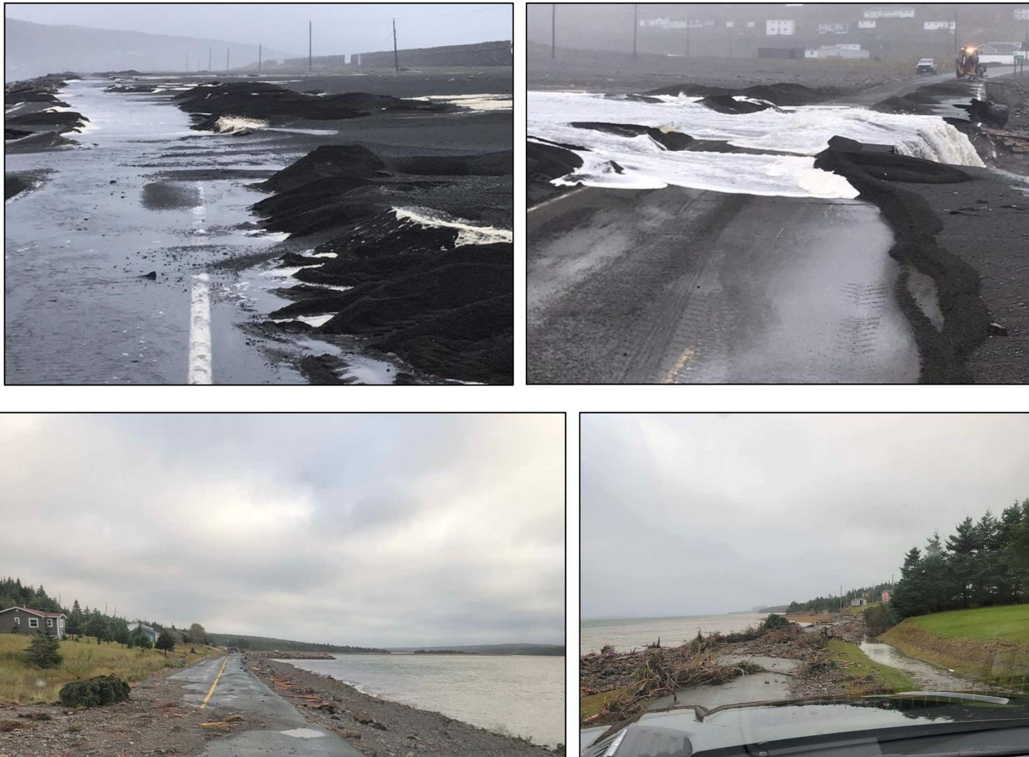
Figure 11. Examples of overwash, damage, and debris along low-lying roads along the south-facing coastline of the Avalon Peninsula in Newfoundland after the passage of Hurricane Larry. The top two pictures are along on Route 90 at St. Vincent's and the bottom photos are of Route 92-10 (Lower Road North Harbour). Photos courtesy of the Government of Newfoundland and Labrador.
