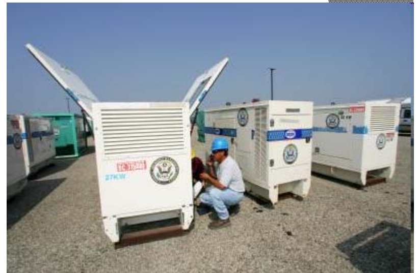
Workmen ready generators to be placed in communities affected by Hurricane Rita. Bob
