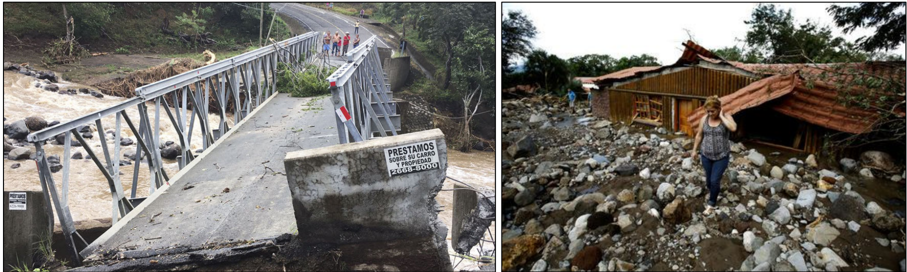
Figure 9. Photo of damage to a bridge (left photo) over the Blanco River, in Guayabo de Bagaces, Costa Rica. Image courtesy of La Nacion. Photo of damage to a home (right photo) caused by a landslide near Guayabo de Bagaces. Image courtesy of Reuters (Juan Carlos Ulate).
